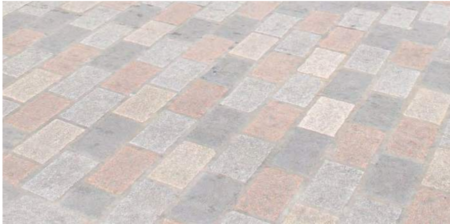
A recessive public realm – a subtle blend of granite in the road
